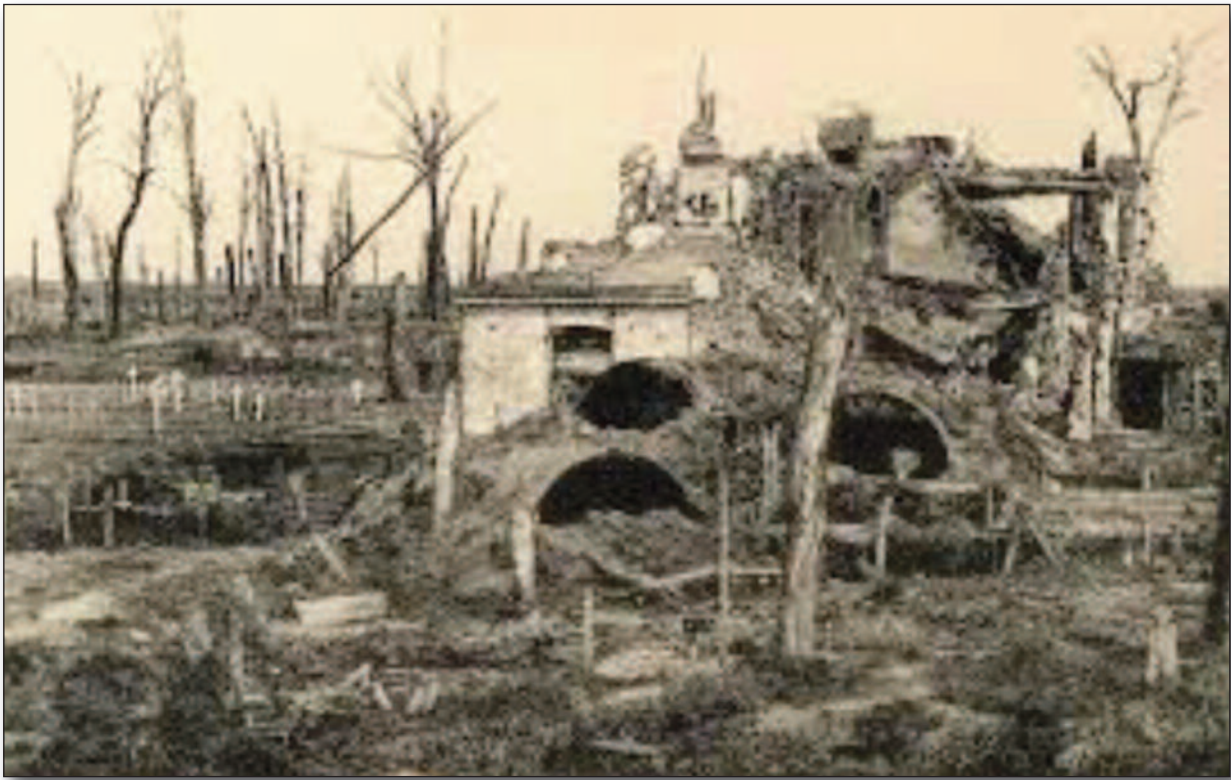
Potijze Chateau first aid post with marked graves in the background taken shortly after the war.
